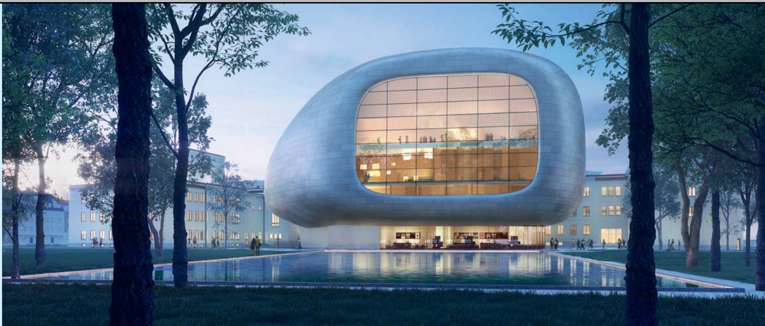
The construction of a new futuristic concert hall in the shape of a violin case in Ostrava city should start within two years Architect: New York atelier Steven Holl Architects and Prague's Architecture Acts ■ Source: City of Ostrava
